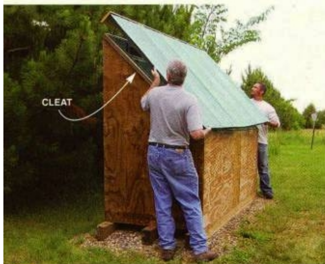
7 With the help of a friend, I set the roof on the kiln. The removable roof hooks over the peak and is secured with screws through a cleat on the side.
